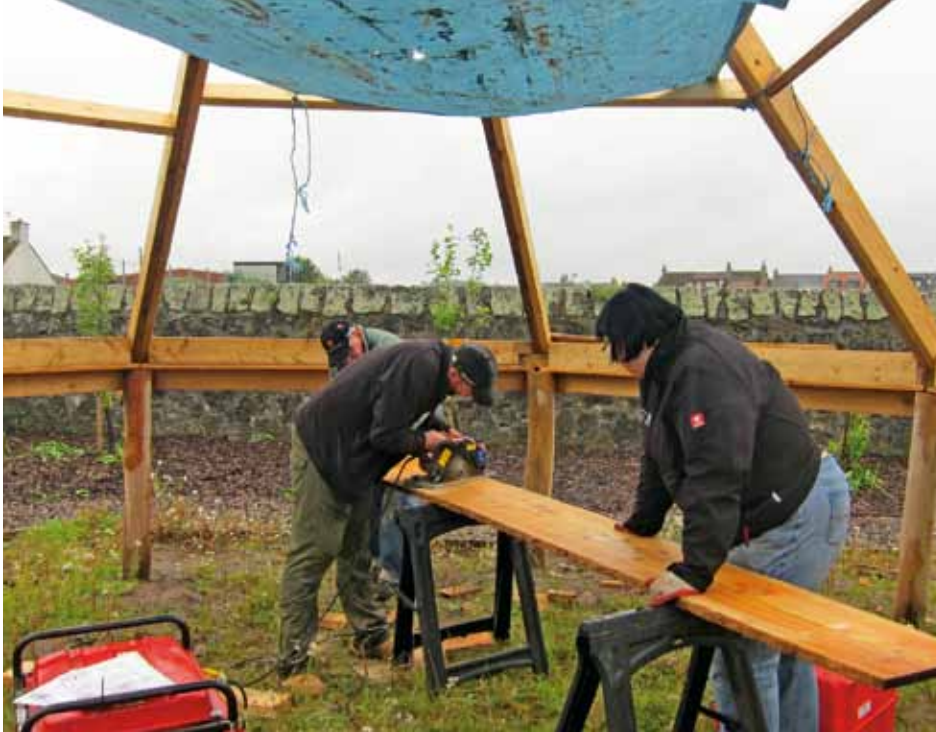
At work, cutting one of the cladding boards for the flatpack classroom
